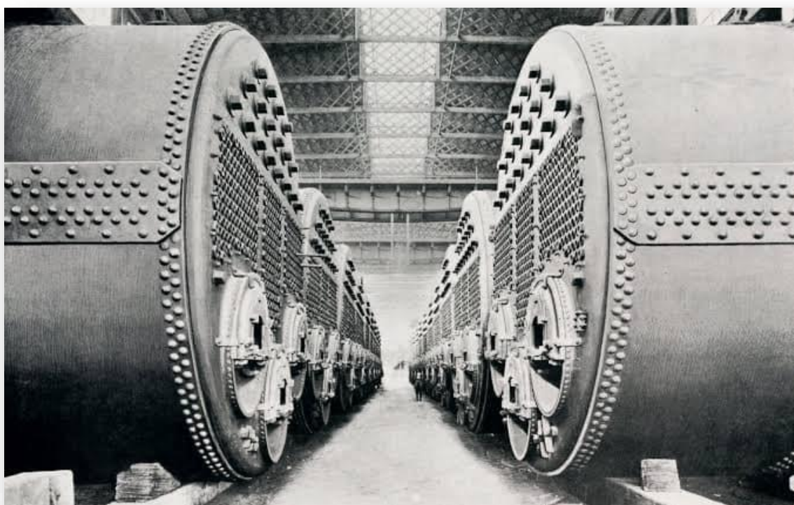
Figure 6: The boilers on the Titanic, photo taken by Mr. Robert Welch.
